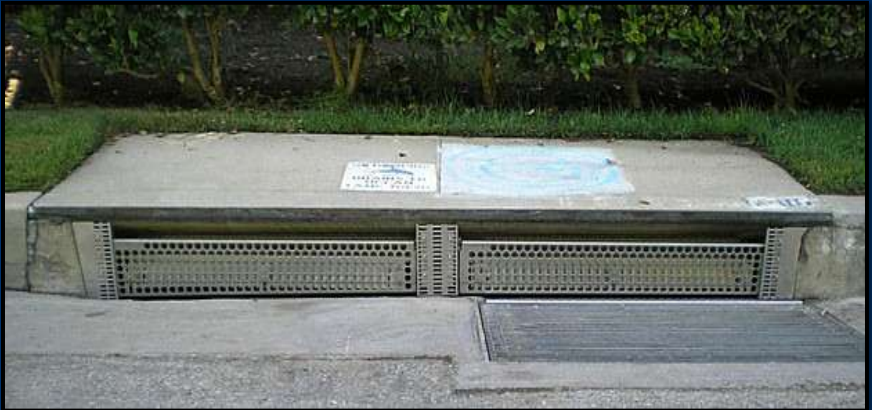
Automatic Retractable Screen (ARS) at inlet throat
