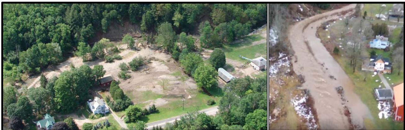
Figure 5: The photo on the left was taken after the 2004 flood event. The photo on the right was taken during the December 2020 high water event. The water can be seen on the 100-year designed floodplain.
