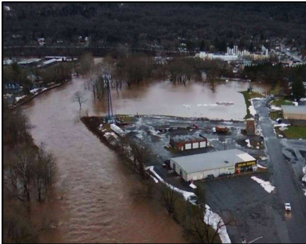
Figure 7: Water Street Floodplain Reclamation Project: December 2020
