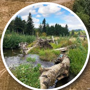
AFTER: Realigned creek with wood habitat structures and thriving riparian vegetation
